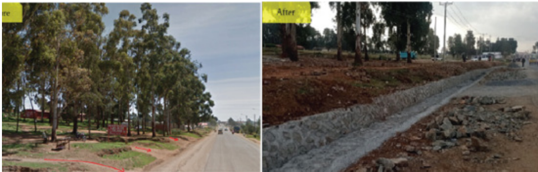
Plate 9-12: On-going construction of storm water drainage along Ol'Kalou – Nyandarua Road
