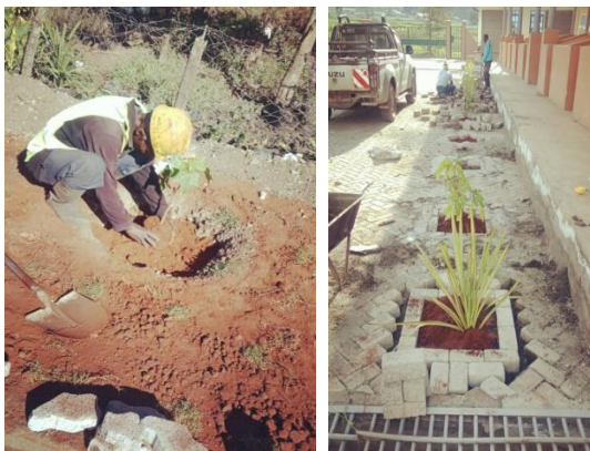
Tree planting (walkway and market area)
