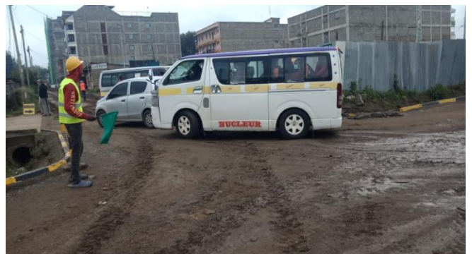
Traffic Control along Estate Roads
