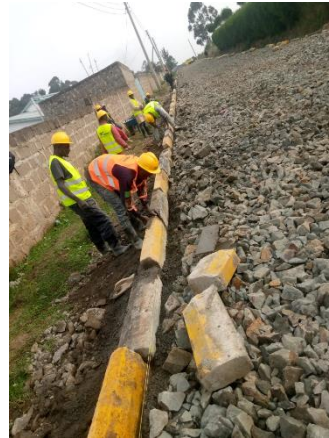
laying of road kerbs
