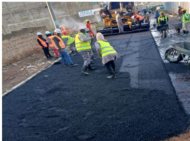
Laying of A/C along Estate Road
